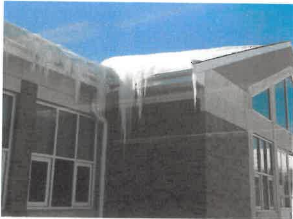
Figure 08: Pitched asphalt shingle roof at 1993 classroom wing.
