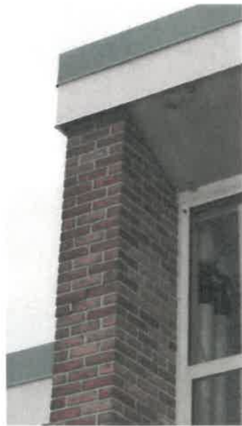
Blade Wall adjacent to Door A3 Note step crack at window mid-height
