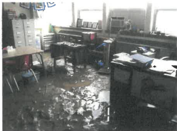
Figure 58: Flood damage at 1956 “Junior wing” as a result of April 2014 water main break.
