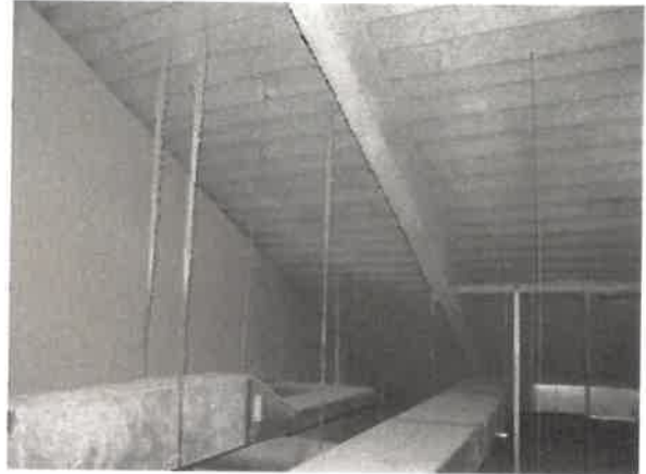
Figure 09: 1993 classroom wing attic space. [Note sprayed on fire-proofing.]
