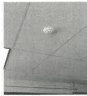
Typical Smoke Detector
