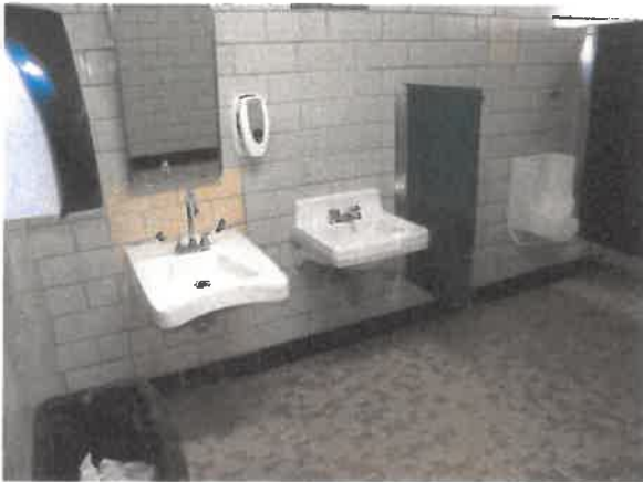
Figure 56: Plumbing fixtures replaced at 1956 toilet room.
