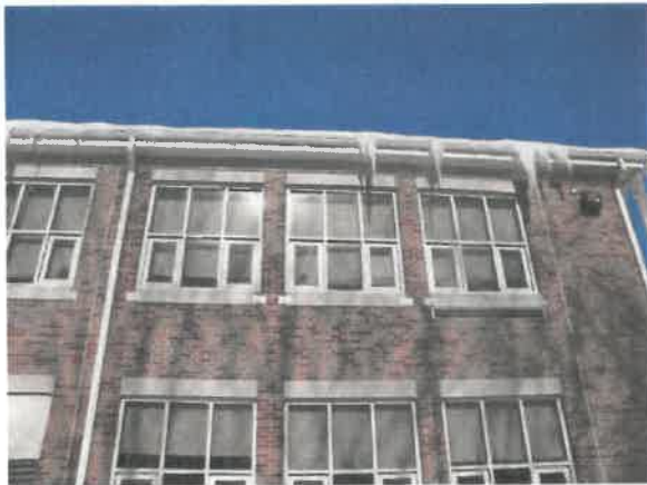
Figure 16: Typical aluminum windows at 1993 classroom wing.
