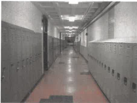
Figure 47: Vinyl asbestos floor tiles at typical 1956 corridors.
