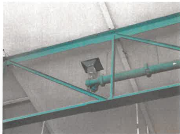
Figure 57: Existing roof drain at 1956 gymnasium.
