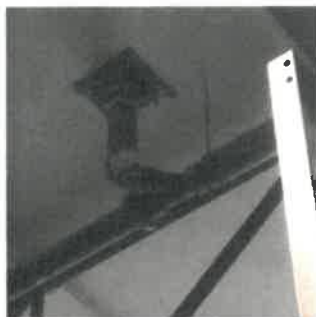
Gymnasium Roof Drain Connection
