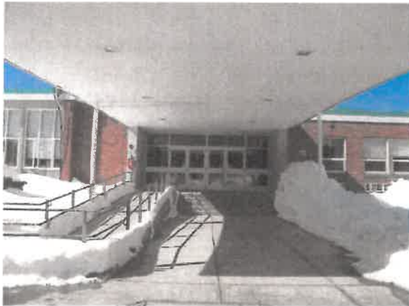
Figure 19: Aluminum doors and frames at main building entrance.
