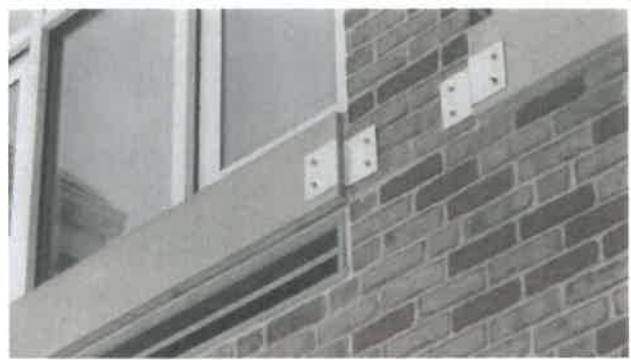
Cast Stone Window Sill Retainer Plate
