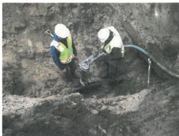
Figure 59: Repair work at April 2014 water main break.
