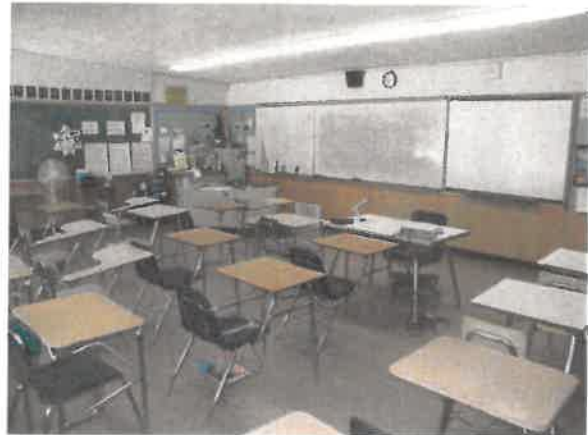
Figure 23: 1956 First Floor classroom.
