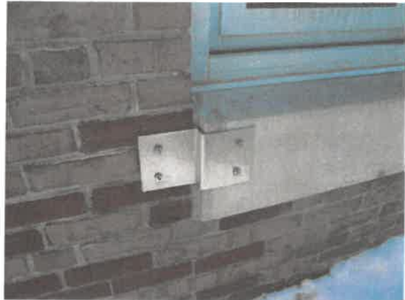
Figure 52: Stainless steel brackets installed to anchor 1993 pre-cast concrete window sills.
