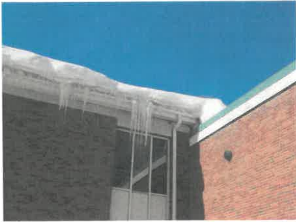
Figure 10: Icicles above egress doors at 1993 classroom wing.
