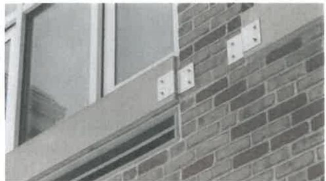
Cast Stone Window Sill Retainer Plate
