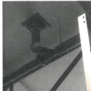
Gymnasium Roof Drain Connection
